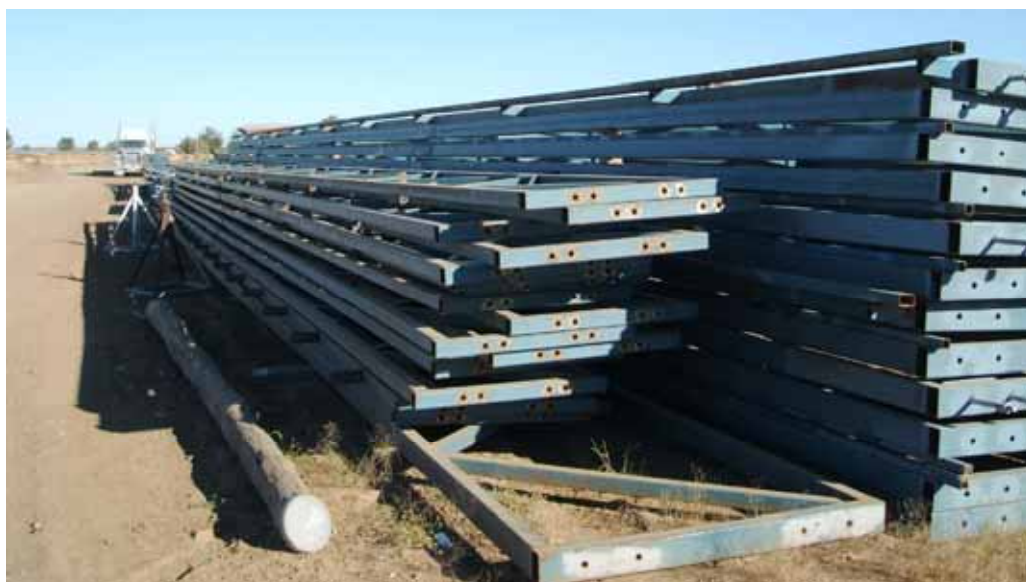
Trusses for factory shed
