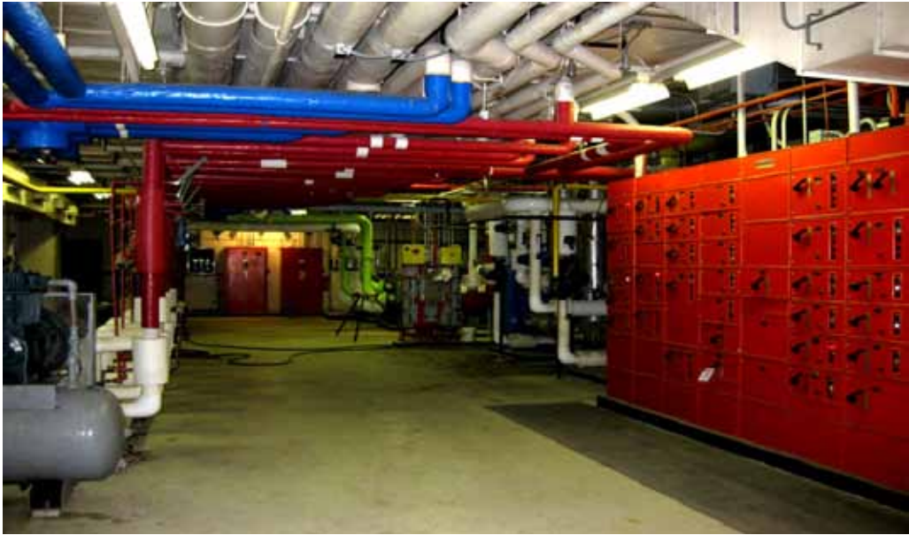
Australian Embassy, Washington. The main electrical switchboards (right of photo) are 40 years old, with parts no longer obtainable. Photo: ANAO
