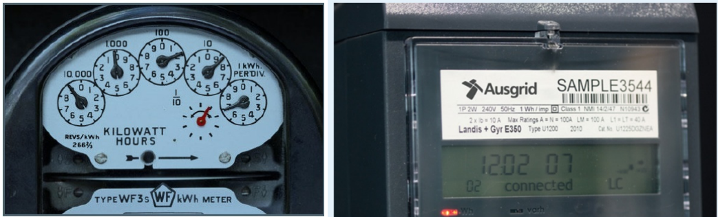
Figure 1.1: Traditional accumulation meter and a smart meter
