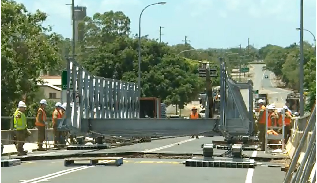
Figure 3.3: Construction of the fixed modular bridge by 2 nd Combat Engineer Regiment
