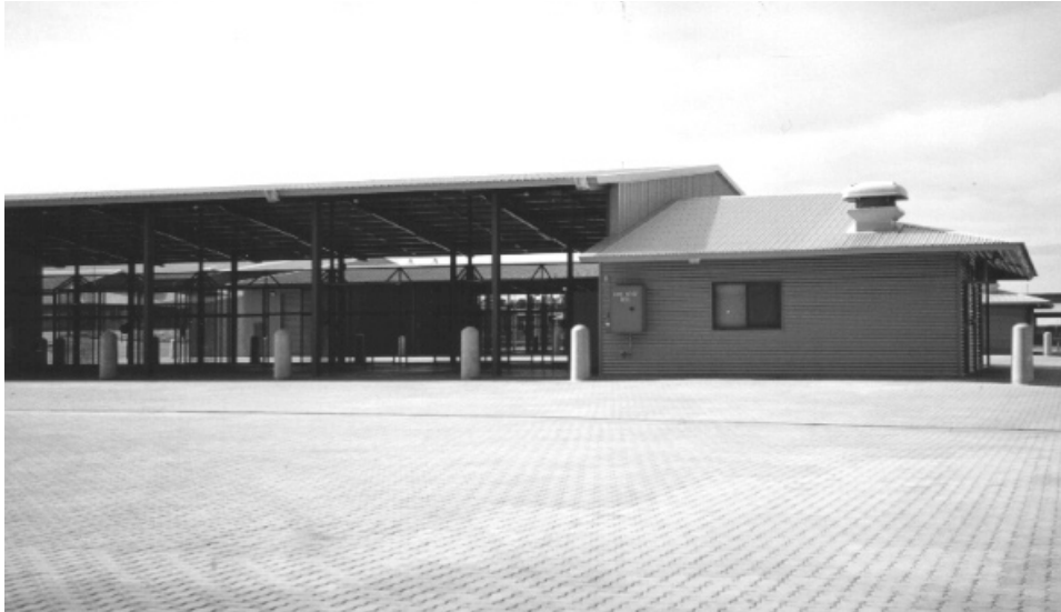
Hangar with reinforced paving, for armoured vehicles at Robertson Barracks
